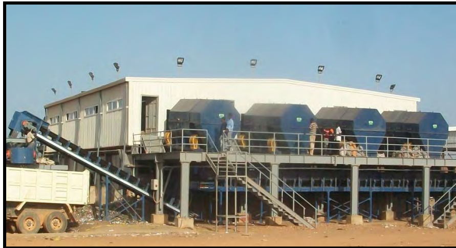
Picture no. (22): Om Dorman municipal solid waste sorting and recycling plant - Sudan
