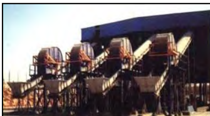
Picture no. (38): Design and construction of MSW recycling and composting plants
