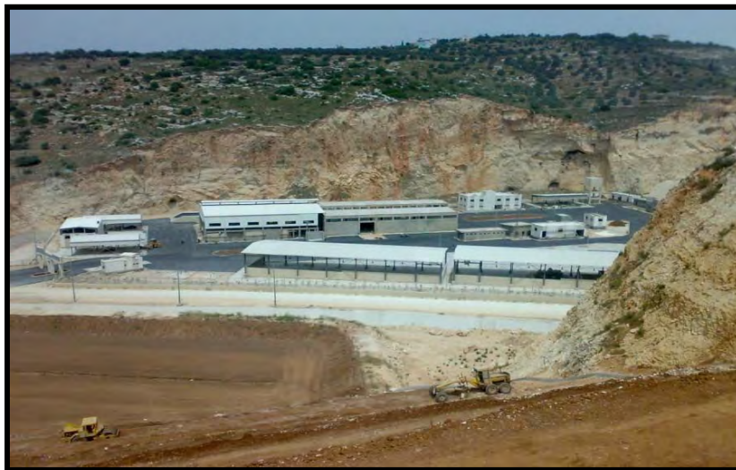
Picture no. (20): Tartous municipal solid waste sorting and recycling plant - Syria
