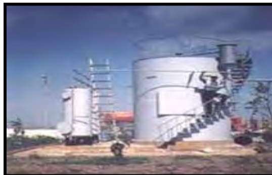
Picture no. (41): Common aerobic composting for treatment of waste resulted from sewage treatments
