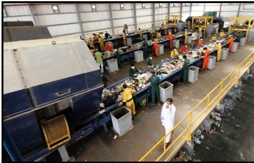
Picture no. (21): Seder municipal solid waste sorting and recycling plant – Jeddah KSA
