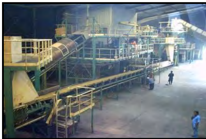
Picture no. (35): EL SAWANY MSW treatment plant - Libya
