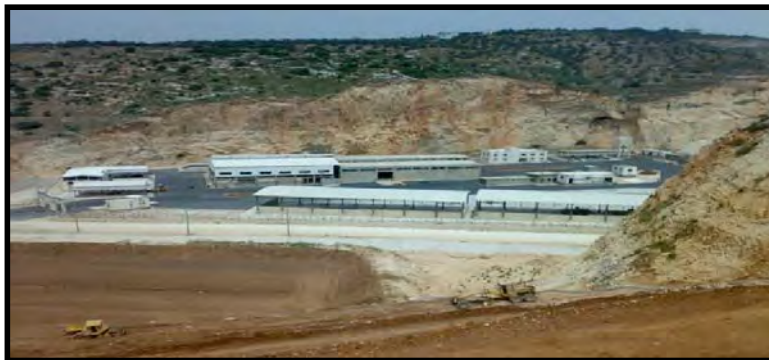
Picture no. (14): Municipal solid waste sorting and recycling plant - Syria
