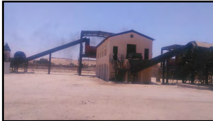
Picture no. (5): Rehabilitation of Sanour Facility
