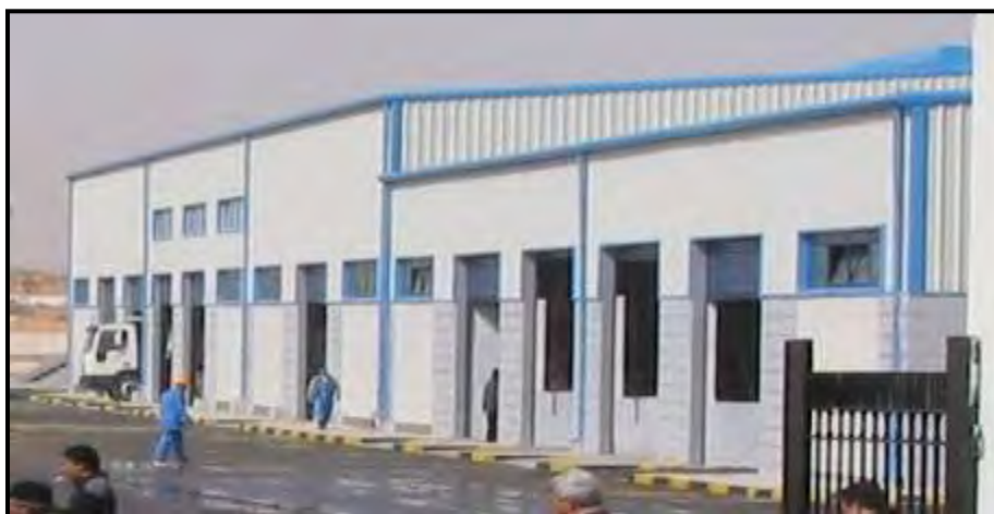
Picture no. (36): Sedy El Sayeh MSW sorting & composting Turnkey plant - Libya
