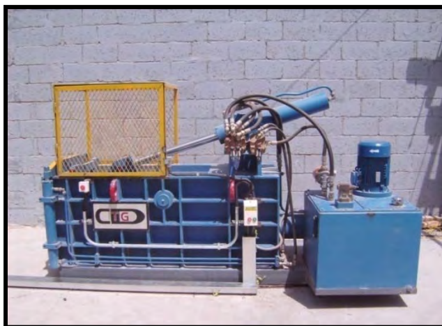
Picture no. (27): El Doha transfer station - Qatar
