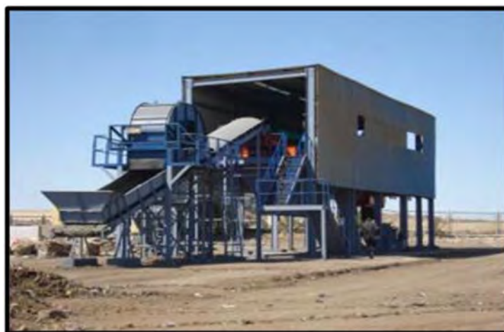
Picture no. (26):Design and construction of MSW recycling and composting plants.
