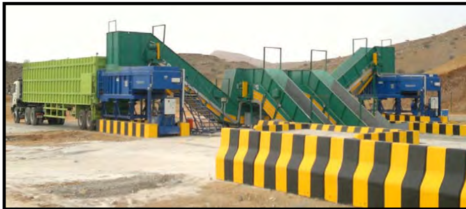
Picture no. (2): Supplying & installing equipment for a transfer station-Oman
