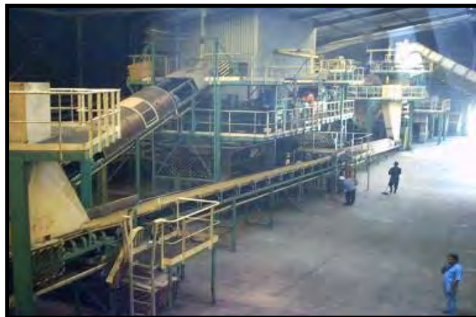
Picture no. (29): EL SAWANY MSW treatment plant - Libya
