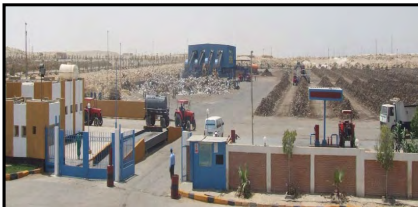
Picture no. (4): Landfilling and processing services for southern Zone in Cairo- Egypt
