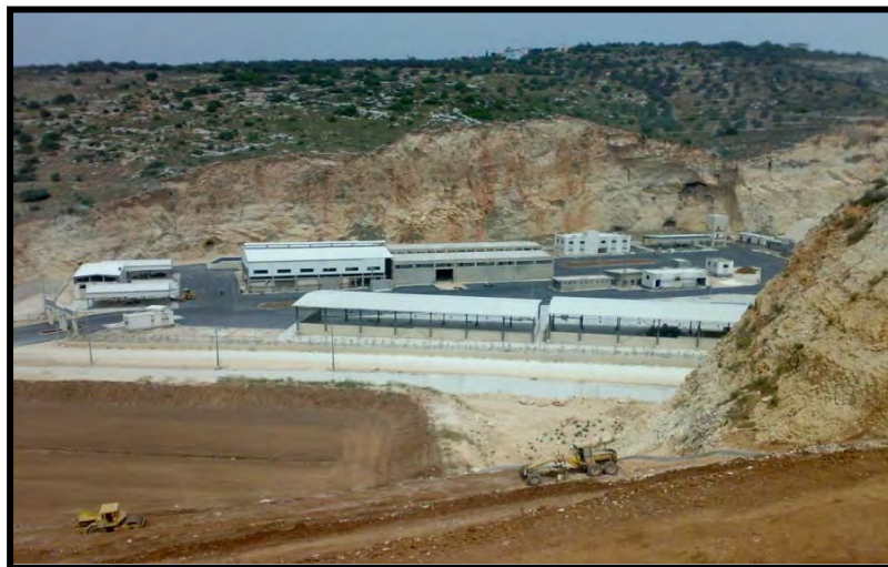
Picture no. (14): Tartous municipal solid waste sorting and recycling plant - Syria
