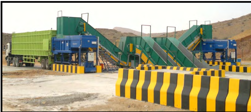
Picture no. (2): Supplying & installing equipments for a transfer station-Oman
