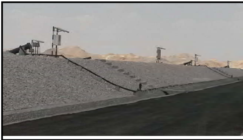
Picture no. (8): Cell Construction
