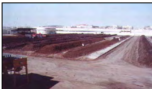
Picture no. (31): Design and construction recycling and composting plant for El Obour Market- Egypt.
