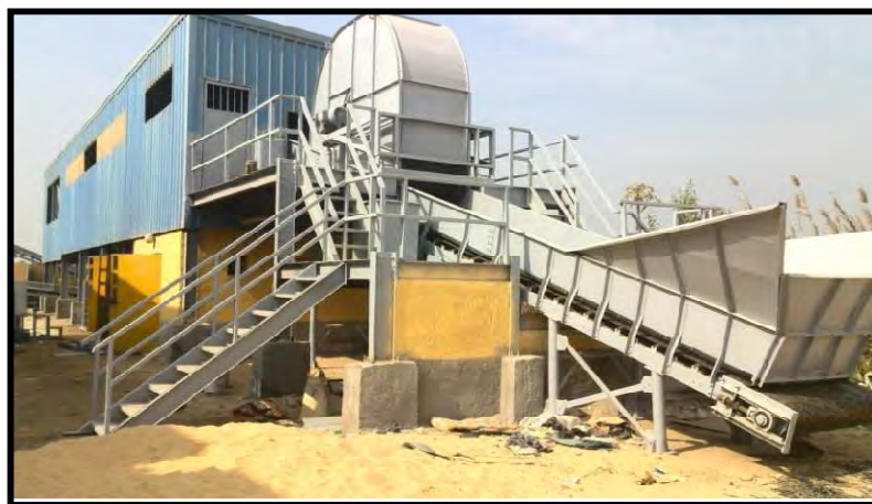
Picture no. (4): Feeding conveyor and bag breaker after rehabilitation process
