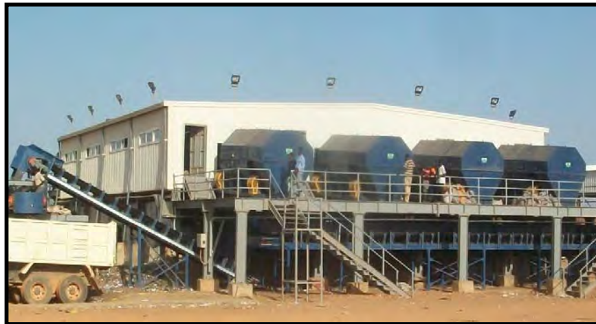
Picture no. (16): Om Dorman municipal solid waste sorting and recycling plant - Sudan
