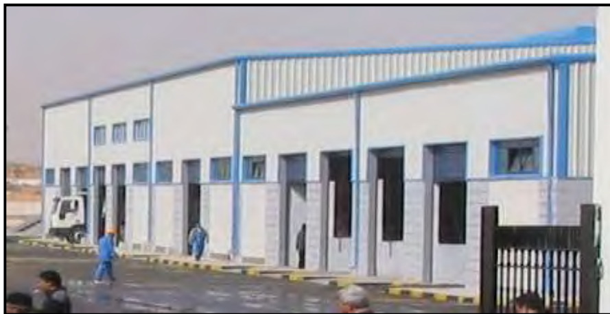
Picture no. (30):Sedy El Sayeh MSW sorting & composting Turnkey plant - Libya
