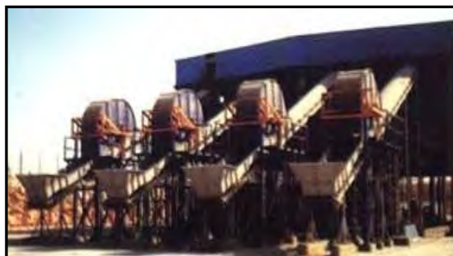
Picture no. (32):Design and construction of MSW recycling and composting plants
