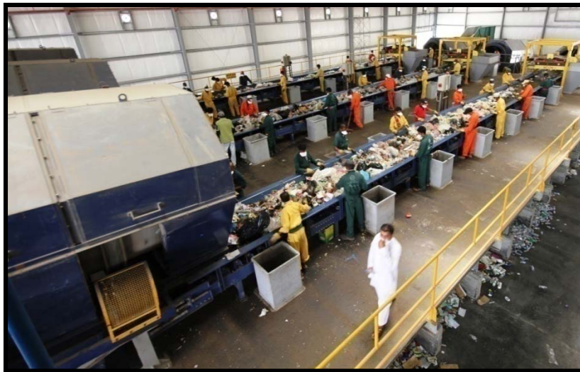
Picture no. (21): Seder municipal solid waste sorting and recycling plant – Jeddah KSA
