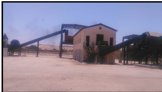
Picture no. (5): Rehabilitation of Sanour Facility
