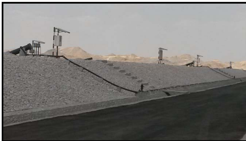
Picture no. (14): Cell Construction
