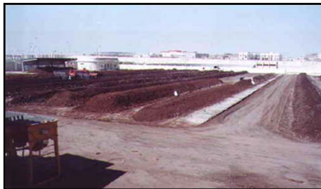
Picture no. (37): Design and construction recycling and composting plant for El Obour Market- Egypt.
