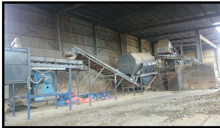
Picture no. (6): RDF Equipment
