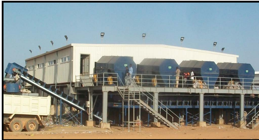
Picture no. (22): Om Dorman municipal solid waste sorting and recycling plant - Sudan
